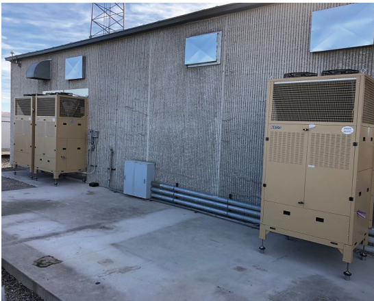
North side of the facility
