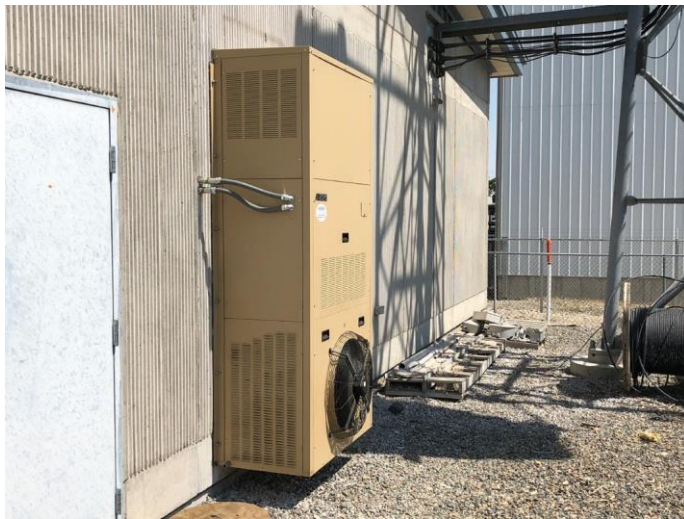
South Side of Helena Data Center
