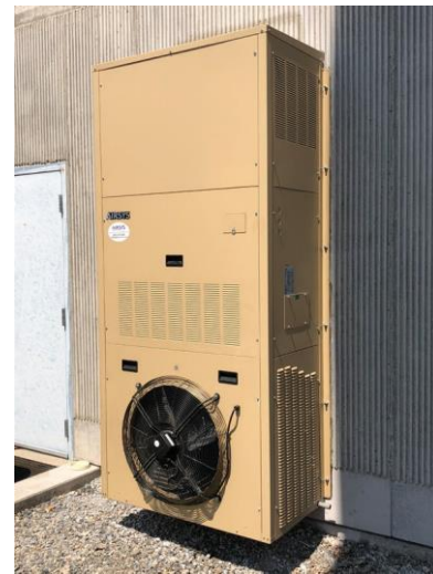
South Side of Helena Data Center
