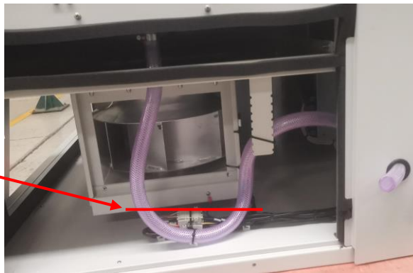
Figure 3-8 Prefill Water to Drain Trap
