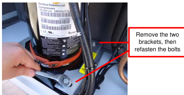
Figure 3-7 Remove Compressor Brackets
