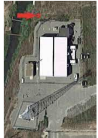
Satellite image of the Laurel facility
