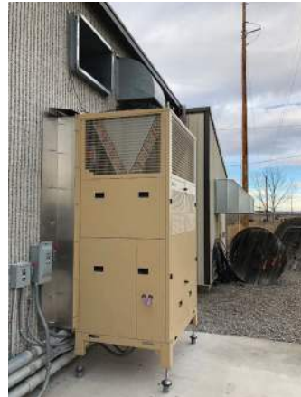
Exterior pad and duct work connections
