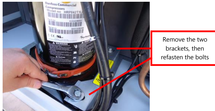
Figure 12: Remove Compressor Brackets
